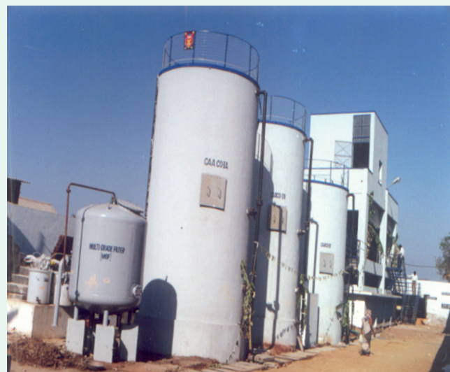
IOR based treatment plant (750 m 3 /day) in a textile industry, Tiruppur, Tamil Nadu
